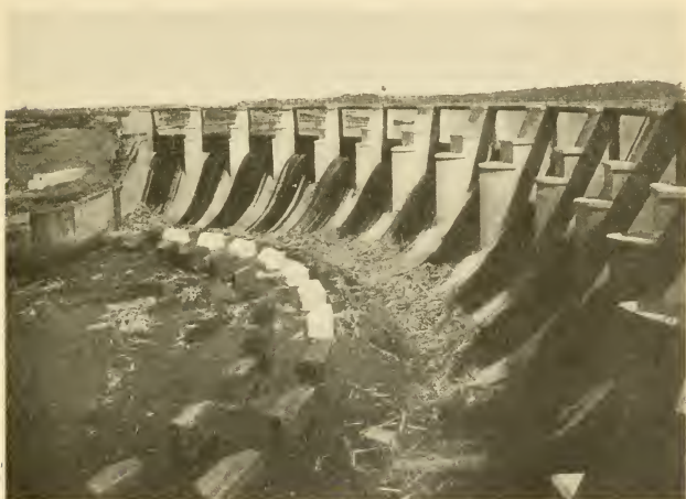
FIG. 4. GATUN SPILLWAY DAM. BAFFLE PIERS IN FOREGROUND. ENTRANCE TO MACHINERY TUNNEL IN DISTANCE.
